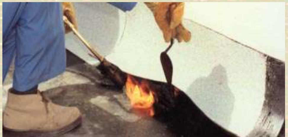
Base Flashing - Proper Torching
