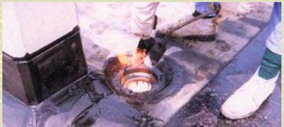
Dressing of Drains.
