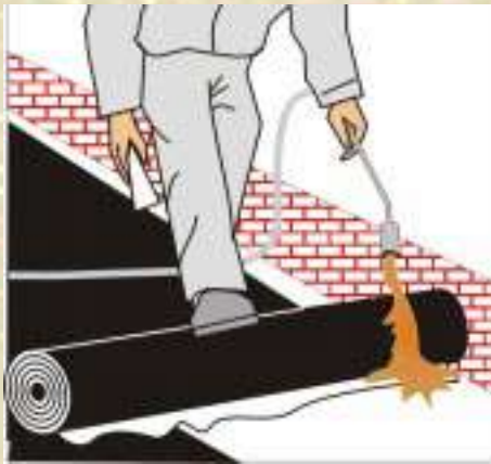
Application of Membrane.
