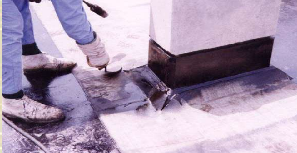
Proper Sealing of Flashings.
