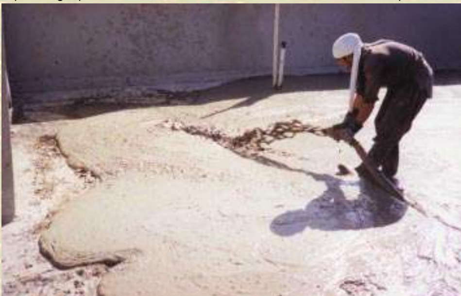
Lightweight Foam Concrete Being Poured.
